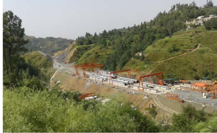
Figure 5 KKH Phase-II (Thakot-Havelian Section)
