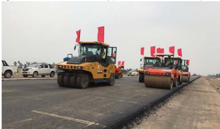
Figure 4 Peshawar-Karachi Motorway (Lahore-AbdulHakeem Section)
