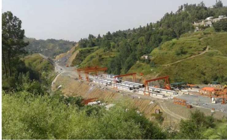
Figure 5 KKH Phase-II (Thakot-Havelian Section)
