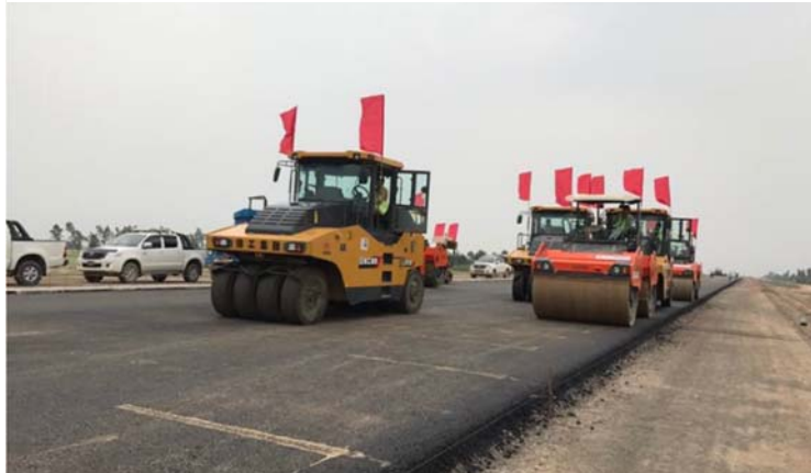
Figure 4 Peshawar-Karachi Motorway (Lahore-AbdulHakeem Section)
